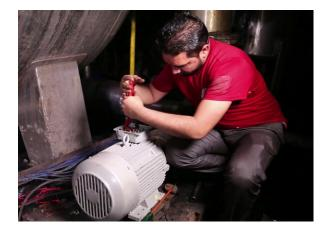
Figure 30: On-site motor replacement
